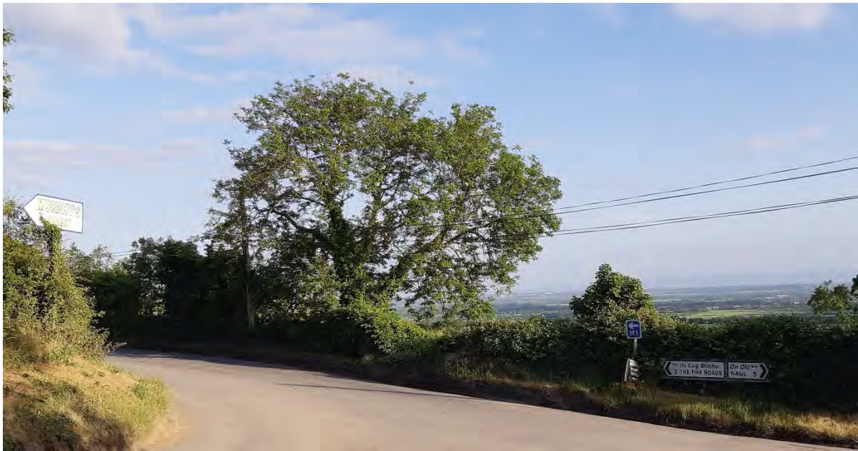
Figure 13-1 LP-1090/ LP-1080 junction looking east
