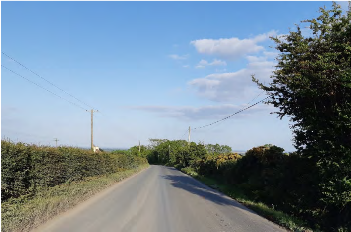
Figure 13-3 Location of new site entrance on LP-1080 looking east
